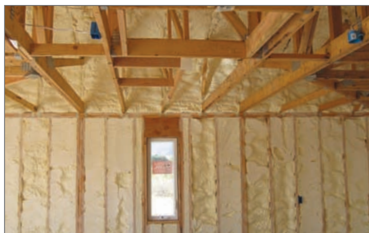
The home with 2 × 6 wood framing was insulated with Icynene foam insulation. This normally-framed home was the only one of three tested that required cooling during the typical peak energy use period.
