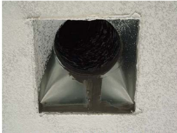
Image 70. Proper sealing around vent cans
